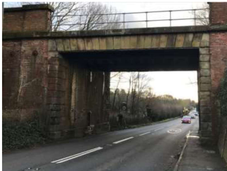
Figure 90: View of bridge from the north. Note the missing section of pipe on the east side beneath the bridge (photograph taken 17 th January 2020).
