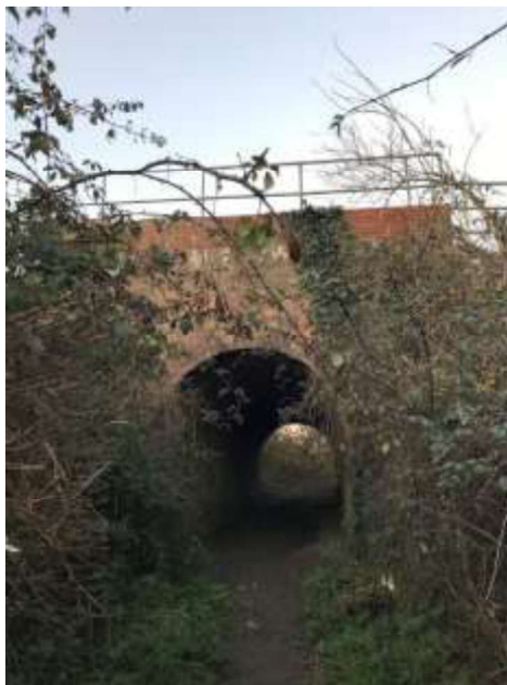
Figure 89: View of bridge from the south (photograph taken 4 th December 2019).
