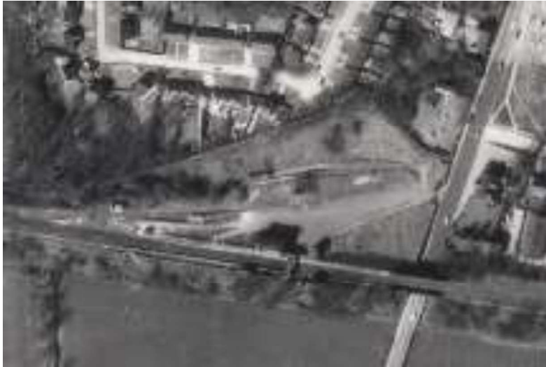
Figure 56: Detail from an aerial photograph taken in April 1971, showing the replacement shelters at the station, as well as the remains of Heasman's wharf to the north and bridge over Eastbourne Road/Station Road (LP24) to the east (HSL/UK/71/37 37/0139 12-APR-1971).
